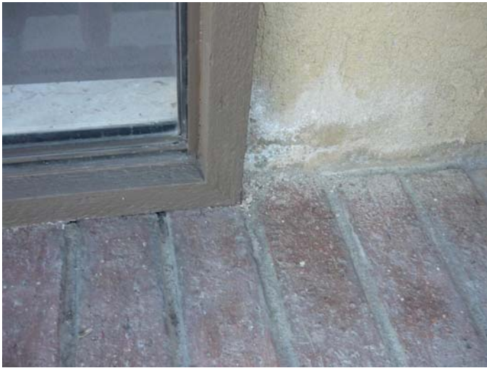
Stucco deterioration.
