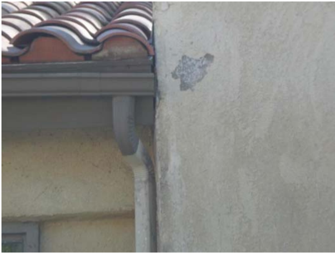
Stucco deterioration.
