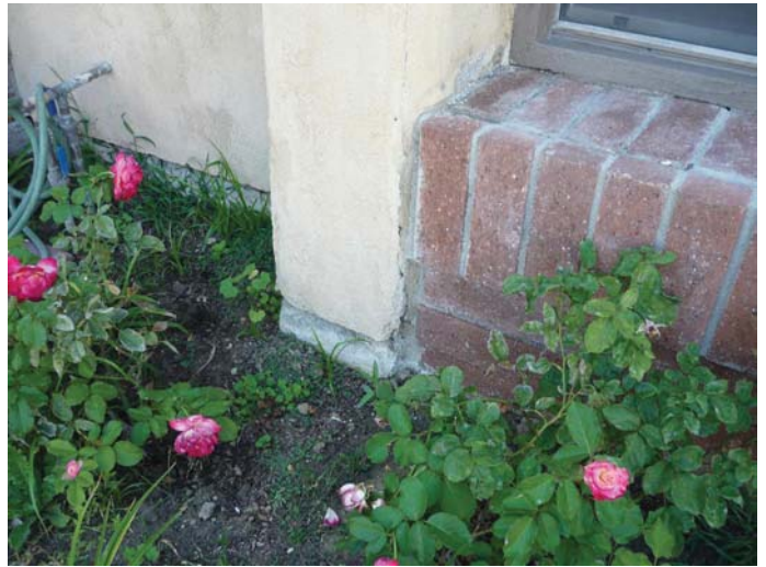
Stucco deterioration.
