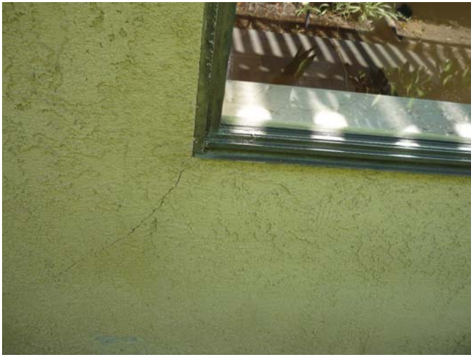
Stucco crack.
